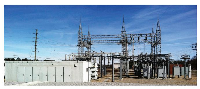
Ibistek is currently engaged in the turnkey construction of a new 161/31.5 KV Substation at Afienya configured in a bus with five bays for the termination of two lines and installation of two 161/34.5KV 100/132 MVA Power Transformers. The project includes civil works, engineering and erections of electromechanincal equipment and transmission towers.
