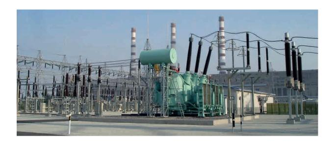
Turnkey construction of a new 161/31.5 KV Substation at Afienya configured in a bus with five (4) bays for the termination of two (2) lines and installation of two (2) 161/34..5KV 100/132MVA Power Transformers.
